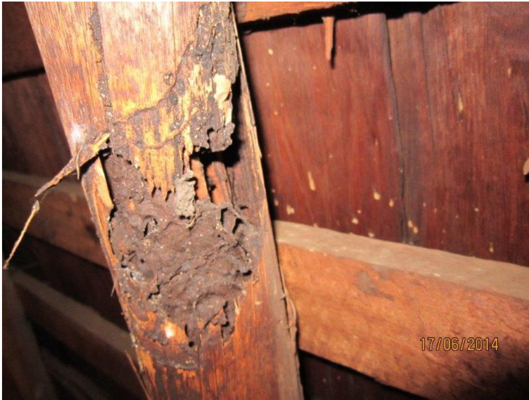
Photo 24 Termite damage
