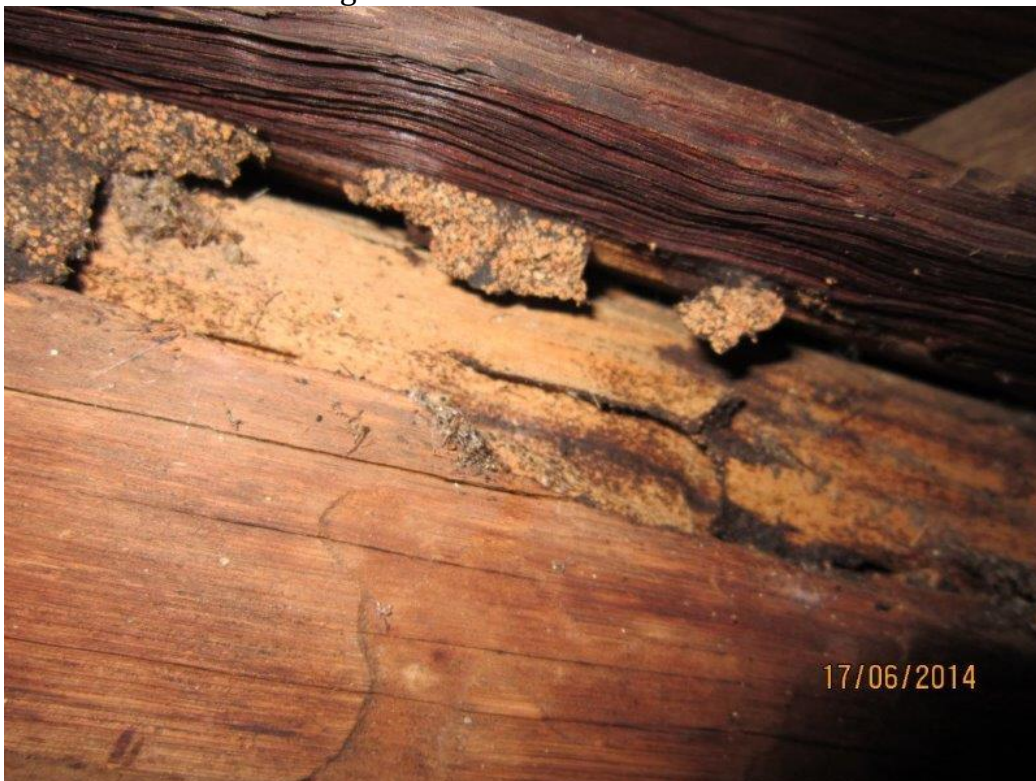
Photo 24 Termite damage
