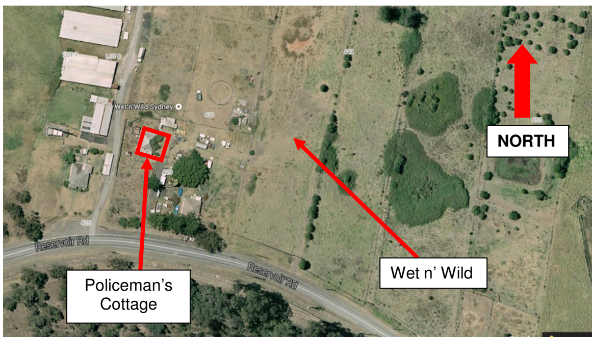
Figure 1 – Aerial view of Policeman's Cottage
